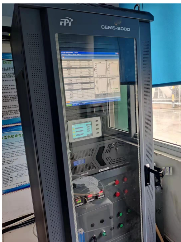
1#RTO 焚烧炉系统在线 CEMS
